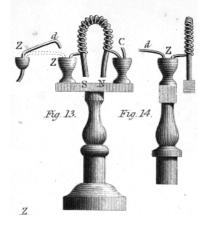
Fig. 1: Sturgeon's electromagnet (1824) showing mercury cup connectors
